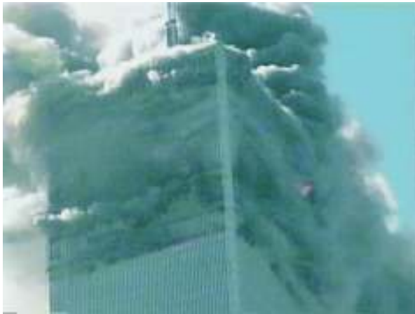
Figure 5-21 The top of the North Tower has dropped a small amount, which means the entire top section has been severed from the base.
