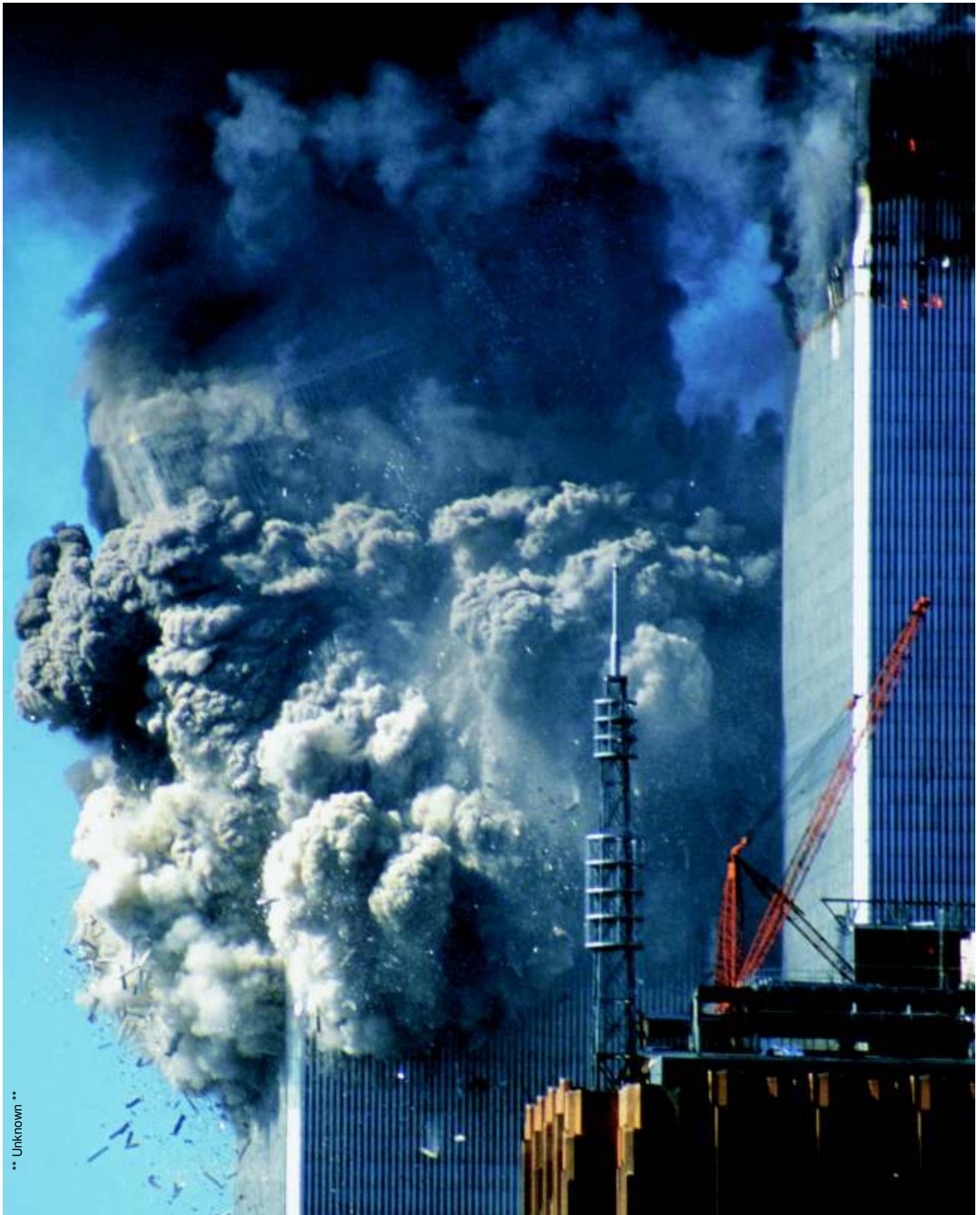
Figure 5-10 The top section of the South Tower has tipped to about 22°. The top of the tower is hanging over the base by about 23 meters in this photo.
