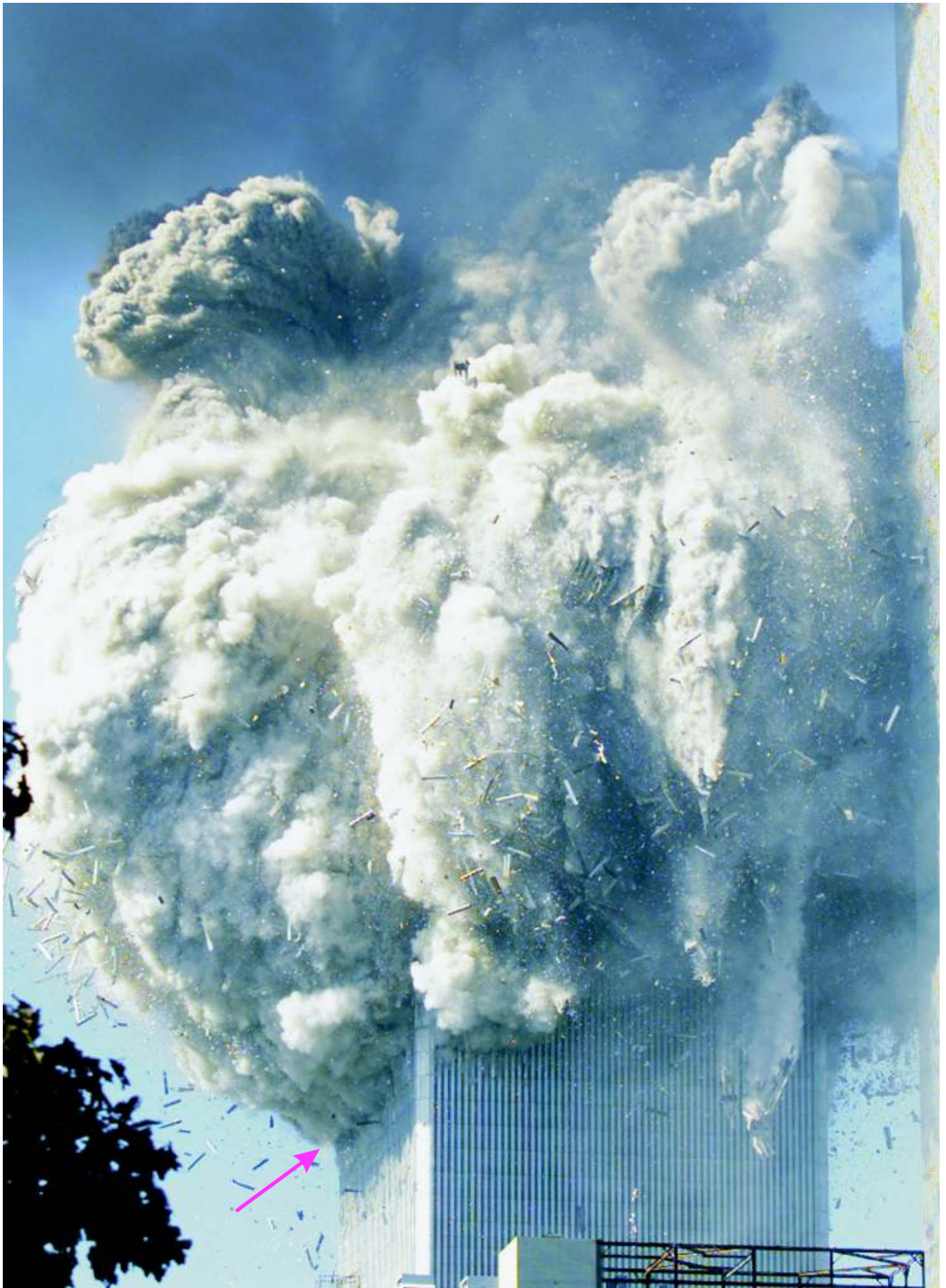
Figure 5-18 The red arrow is pointing to the perfectly horizontal base of the dust cloud. The significance of the horizontal base will be discussed in Chapter 7
