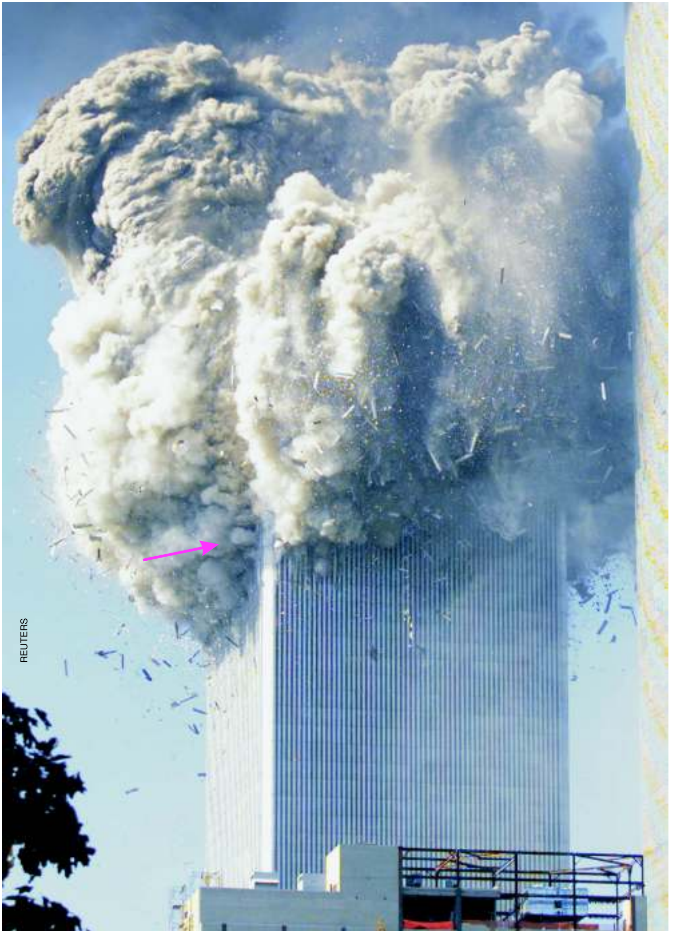
Figure 5-16 The red arrow is pointing to puffs of dust. The significance of the dust will be discussed in Chapter 7
